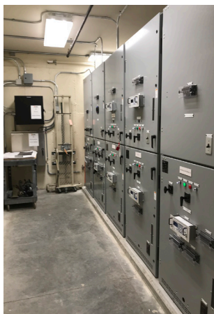
Main Switchgear
