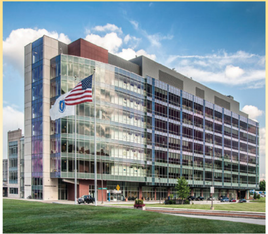
UMASS Medical Center, Worcester
